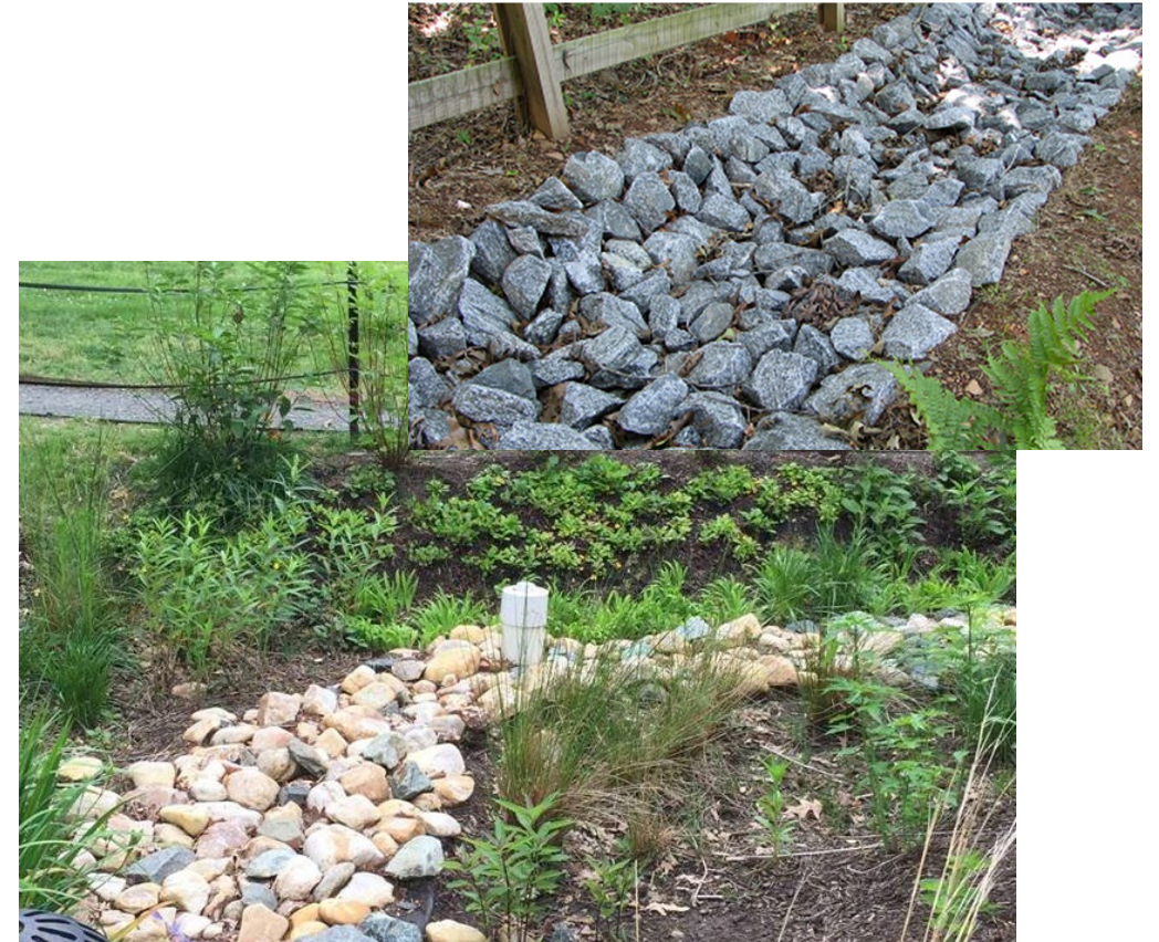
(Examples of rock-lined drainage swales)
